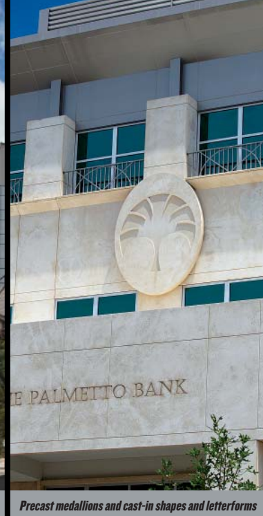
Clever use of reveals and joint detailing hides panelization
