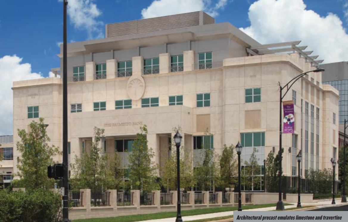
Precast medallions and cast-in shapes and letterforms
